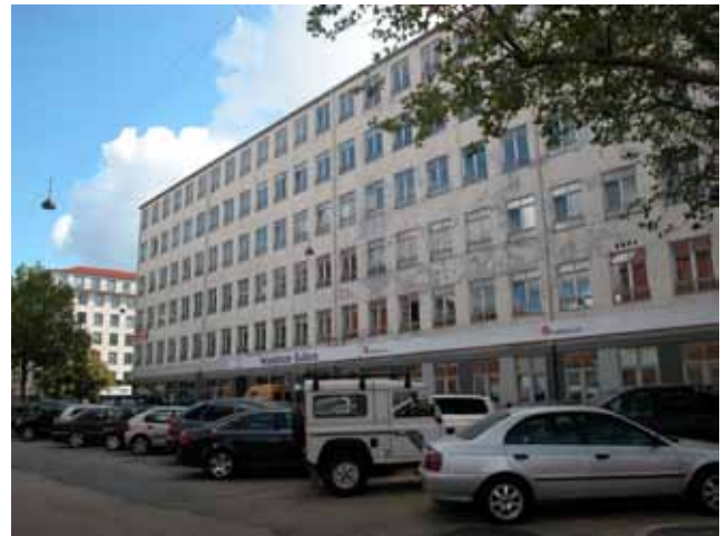
Facade mod Borgergade ("Borgergadehus").
